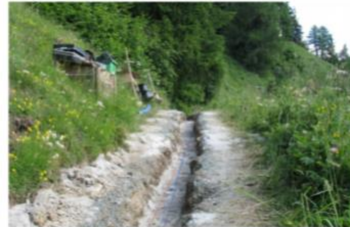
Figure 9. Trench with fiber optic cables installed
